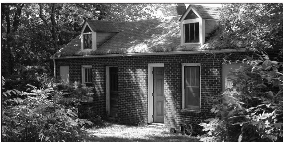
The Foundation acquired the lot and brick building, built by A. S. McNeese in 1942, located behind the OSS. It is part of the original property but not purchased until 2003, made possible by substantial assistance from our neighbor, Security Bank. It is used during our school tours and for storage.
